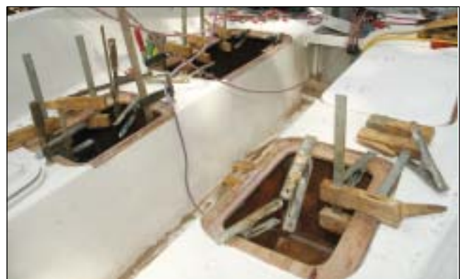
Retrofitting the new hatches.
