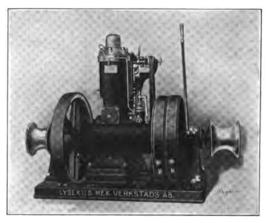
FIG. 354.—Direct-coupled Skandia Motor Winch.
