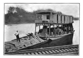
FIG. 269.—Stern Wheeler, with two Decks driven by Remington Engine.
