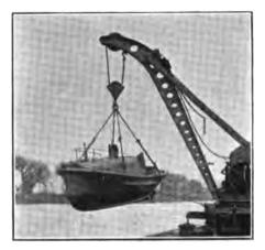
FIG. 283.-Motor Launch for carrying on Steamers' Decks.
